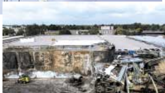
Put to the test in The Netherlands: This wall of Paroc Fire Proof Panels stood virtually unscathed after the building in the foreground burnt down.
