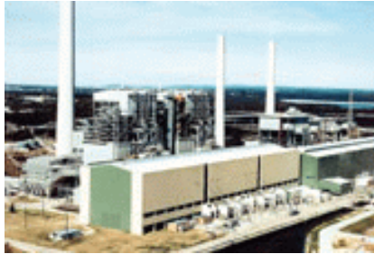
HM Low Profile Ventilators, Vales Point Power Station, Australia
